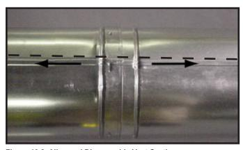
Figure 10.8 Align and Disassemble Vent Sections
